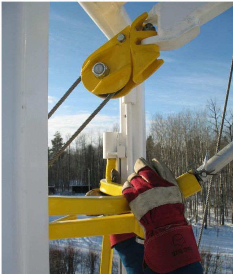
2.13.8 Guide the two docking pins into the docking station's magnetic receiver tubes.
