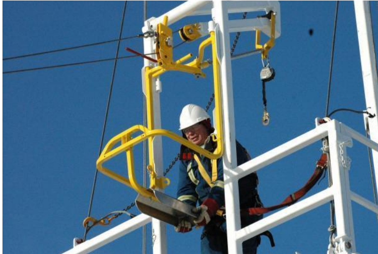
2.13.7 Guide the shuttle into the receiving tracks on the archway.
