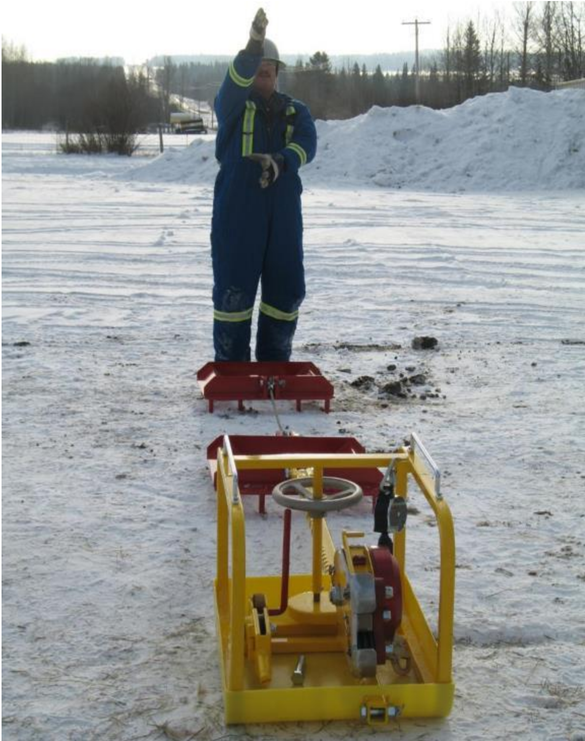
2.5.12 Align the Magnegress system to the top anchor point.
