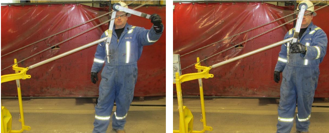
2.12.2.4 Install the pivoting fall arrest trolley by rotating the arm around both cables.
