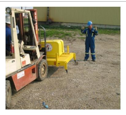
2.6.2. Position the front of the anchor approximately in line to your mark on the ground.
