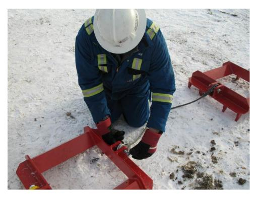
2.5.2. Position the secondary Bear Claw park-on anchor so it attaches to the joiner cable & install joiner cable bolt through two ears capturing the cable between them. Install nut & safety pin.
