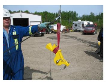
2.3.1.3. Fasten a hoisting sling securely around the docking station, attach the assembly to the winch & tag line. (If mounting the docking station without the cable proceed to 4.2.3.)
