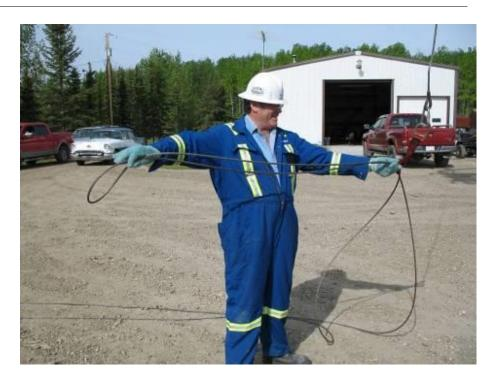
2.3.2.3. Fasten a hoisting sling securely to the cable leaving approximately 6 ft (2.8 m) of tail.
