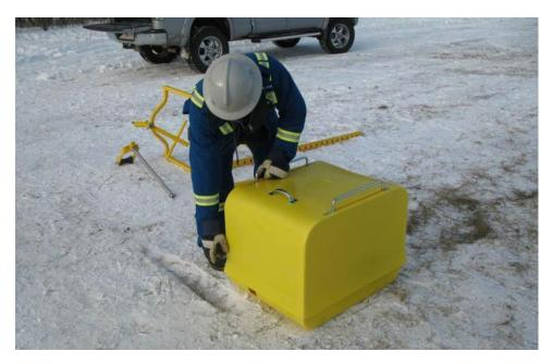
2.4.3. Position the back of the Magnegress frame approximately in line to your mark on the ground.
