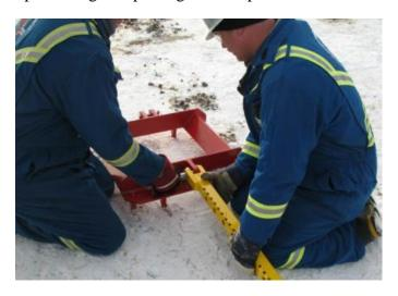
2.5.1. Position the Bear Claw park-on anchor so it attaches to the tension link & install anchor bolt through tension link. Install nut & safety pin.
