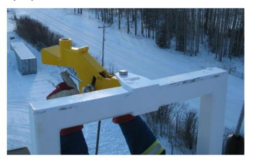
2.3.2.14. Flip down the sheave gate into its closed position & install the safety pin.
