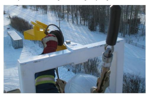
2.3.2.12. Insert sheave inside the 180° back bend & line up the flats on the sheave shaft to the slots in the docking system.
