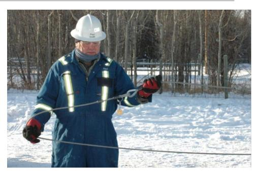
2.7.3. Keeping the cable separated grasp cable firmly & walk towards the desired anchor position.
