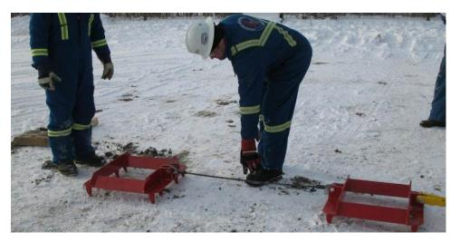
2.5.3. Drag the rear Bear Claw anchor back away from the front anchor until the cable becomes taut.
