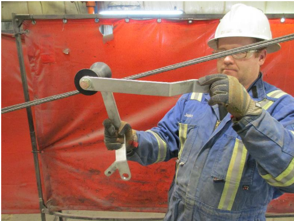
3.13.4. Install the pivoting fall arrest trolley by rotating the arm around both cables.
